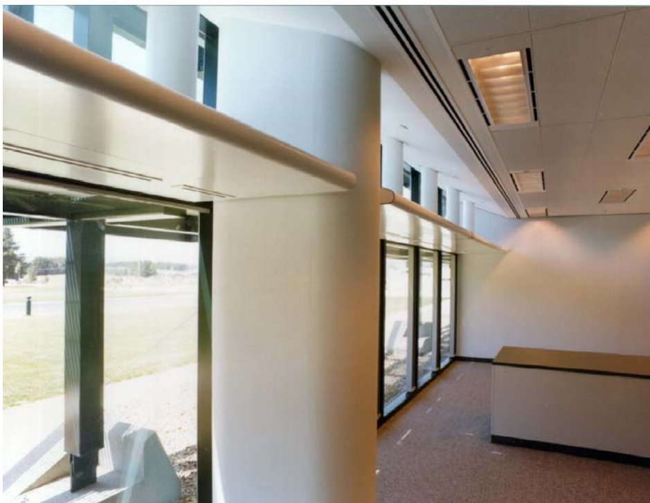
Figure 8. A light shelf and sloping ceiling is used to reduce the contrast between the ceiling and the glazing thereby allowing more daylight to enter the space without creating gloom. The end wall is lit to increase the luminance of the wall. The glass below the shelf has tinted glass to reduce the sky glare while the upper section of glass is clear to maximise the daylight 6
