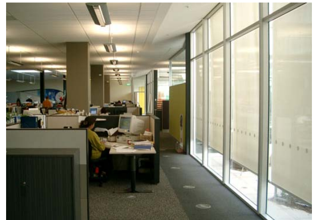
Suspended luminaires, and external screens on courtyard windows.
