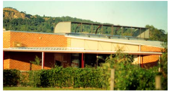
View from northeast, showing skylight and window shading.
