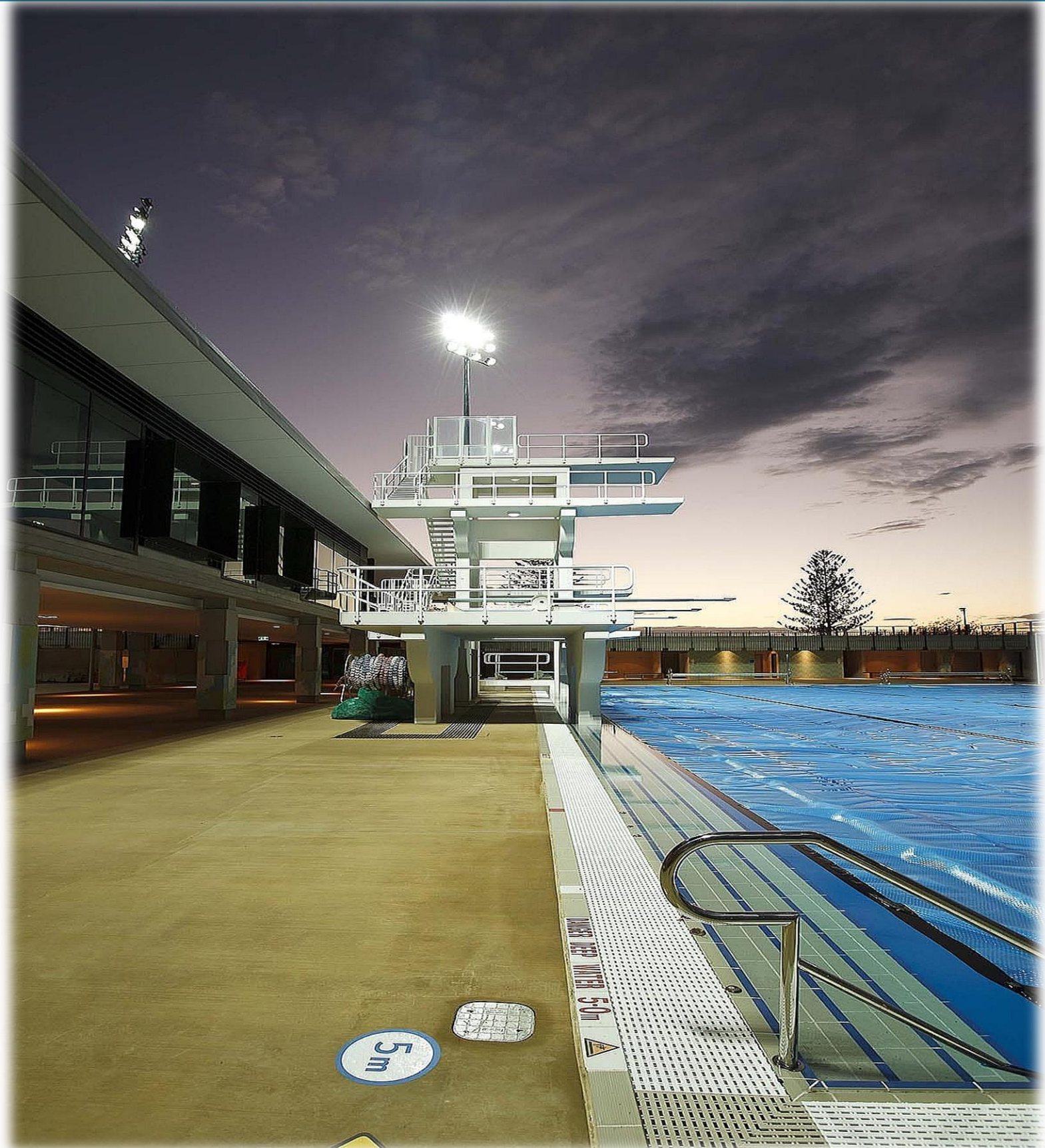
Gold Coast Aquatic Centre, Photo is courtesy of WATPAC
